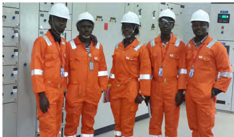
The Participants at the Motor Control Center (MCC) of the Midwestern Oil and Gas Production Facility, Umusadege, Kwale, Delta State.
