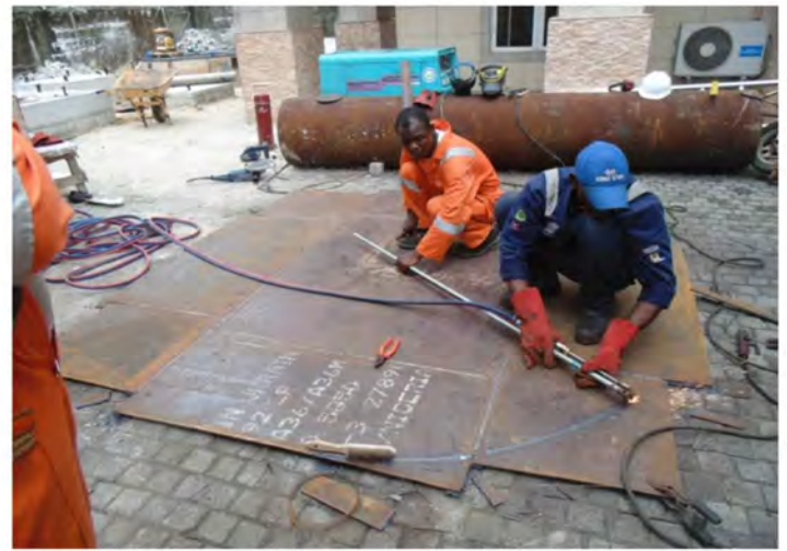
Tank Base Plate Cut-Out
