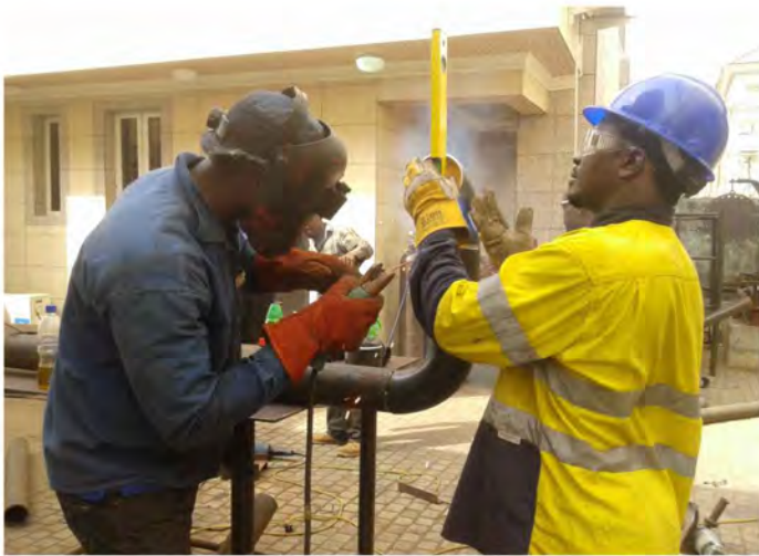
Plant Foundation Setting
