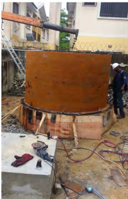
Storage Tank Shell Positioning
