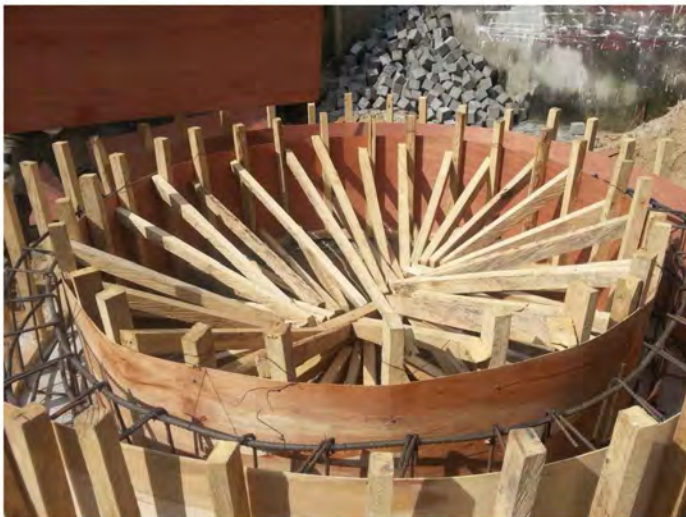
Storage Tank Ring Wall Set-Out
