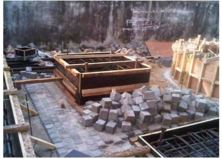
Plant Foundation Setting
